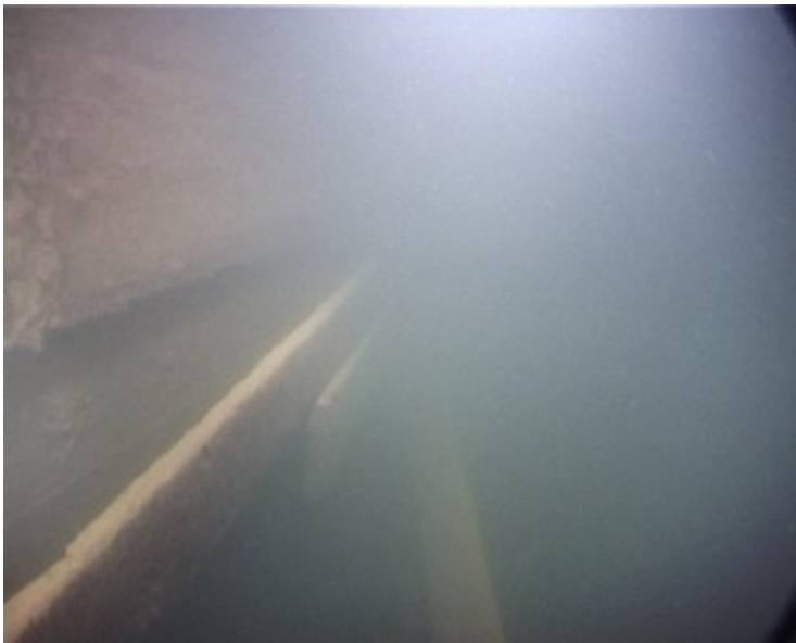
Picture 48. Loose planks on the port side below the main wale in the mid-ship area (view from the bow towards the aft). Photo by P. Raasakka & J. Kaasinen.
