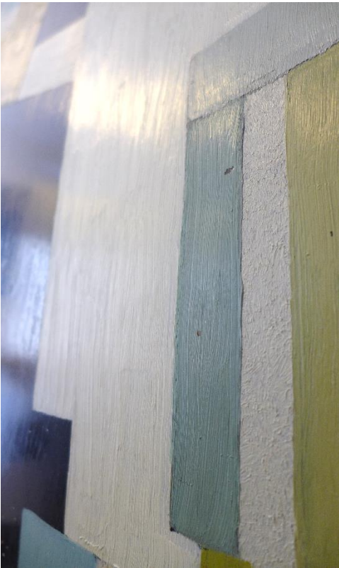
The different textures on the color board created by the brush strokes and technique. This picture presents the textures of the board located in Paimio hospital.
