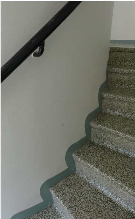
The stairs climbing around the chimney of C-wing.
