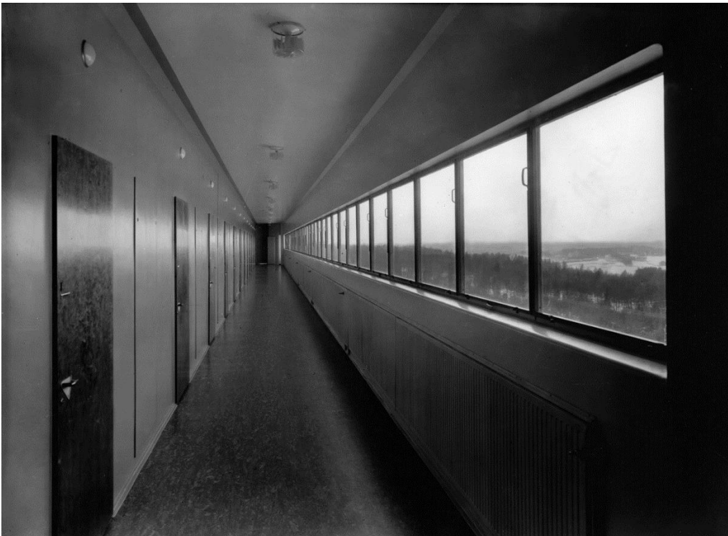
Ward corridor of 5th floor presents the original look and confining of color. Notice the corners of walls and ceiling, the original radiators, laquered doors and linoleum flooring. AAM. Sign. 50-003-328.
