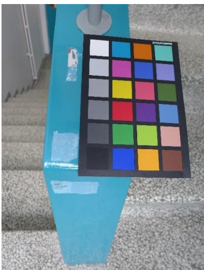
The staircase with panoramic lift, in the west end of the wards.
