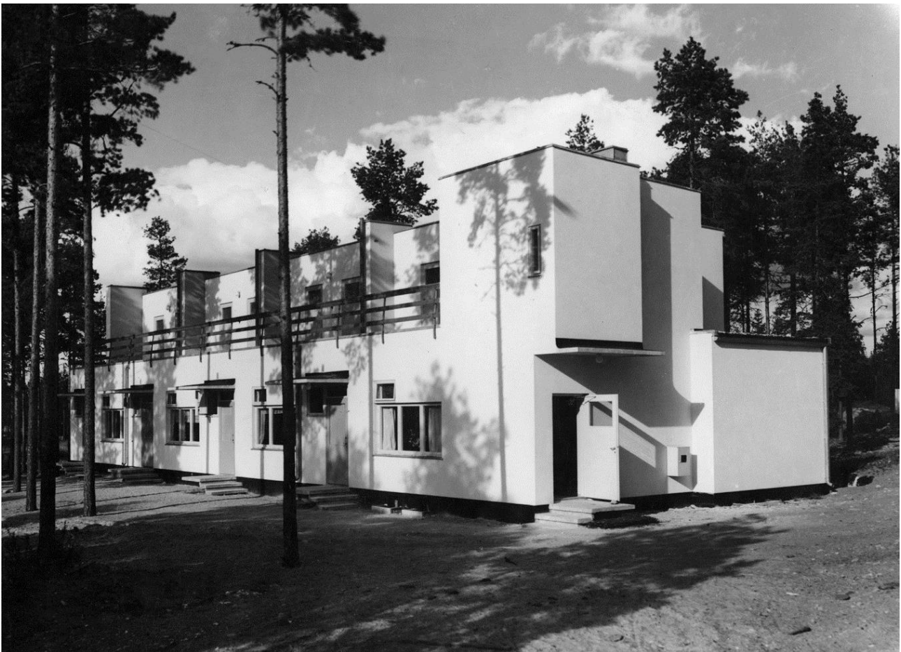
Staff apartment building soon after its completion. AAM Sign. 50-003-432
