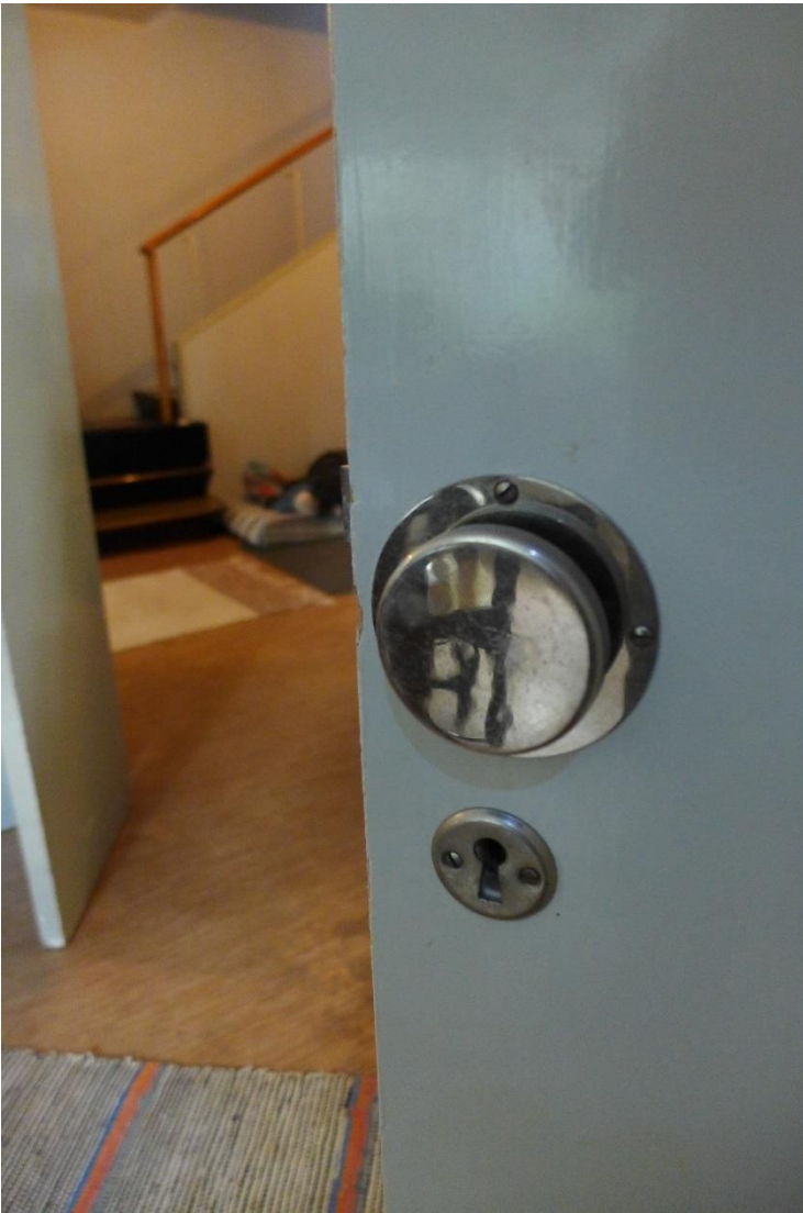
A detail of the original sliding door between the lobby and living room.
