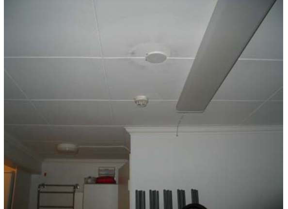
Katto on levytetty.
