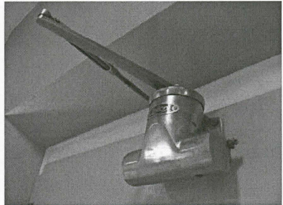
Hissinoven ovipumppu, Abloy.
