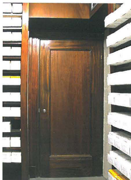
Ovi 2: Mahonkinen umpipeilinen kehysovi.
