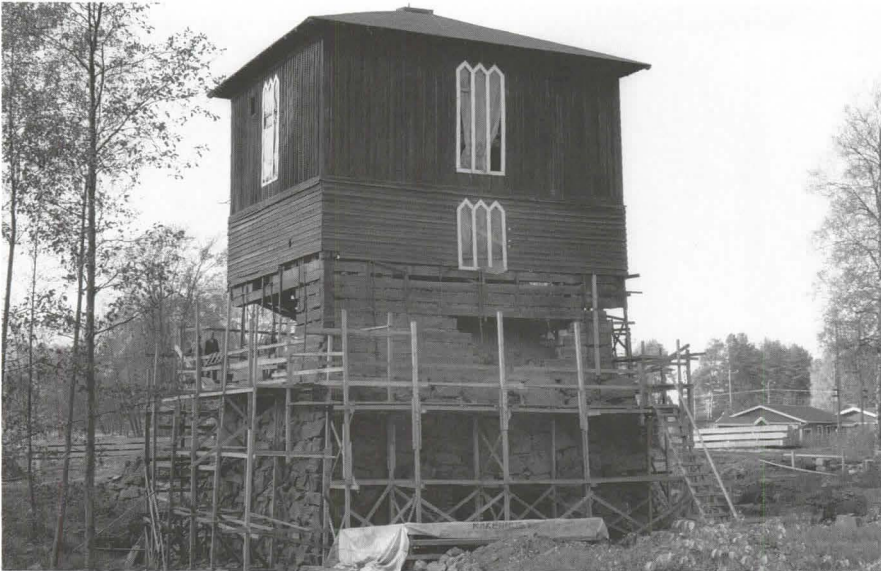
Osia multahirsistä on jo poistettu, yläosa on nostettu terästukiristikon varaan. Part of the timber cladding has been removed, and the upper part of the blast furnace is supported with framework of steel members.
