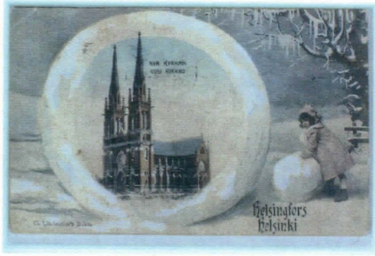
WHAT IS THE CONDITION OF THE FAÇADES ?
