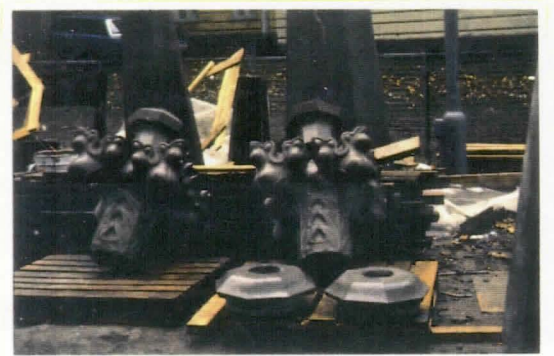
NEW PARTS OF THE FINIALS OF THE TRANSEPT PINNACLES.
