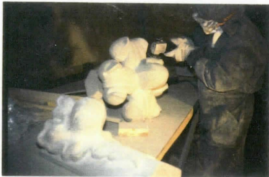
FINISHING A FINIAL BY GRINDING
