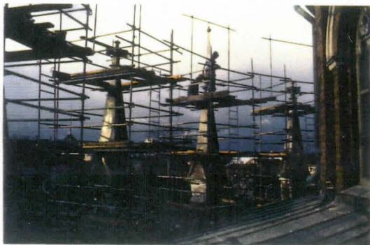
REPAIRING AND RENEWING THE PINNACLES OF THE CHOIR.
