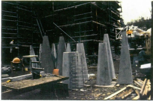
CASTING THE NEW PINNACLES ON WORKING SITE. THE "CHURCH CONCRETE" DEVELOPED BY FESCON OY FIRM WAS USED.
