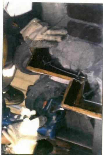
ADJUSTING A DISPENSABLE PLASTER MOULD AND REINFORCEMENT TO A CORNER
