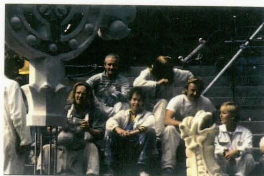
THE WORK IS OVER ! THE RING CROSS IS READY TO BE LIFTED UP .
