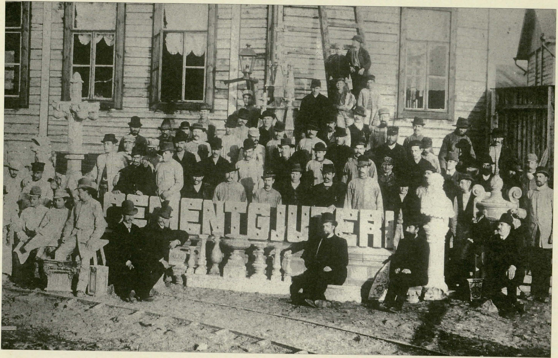
WORKERS OF "Helsingfors CEMENTGJUTERIET" CASTING WORKS WITH CAST CEMENT ORNAMENTS FOR THE CHURCH OF ST JOHN.
