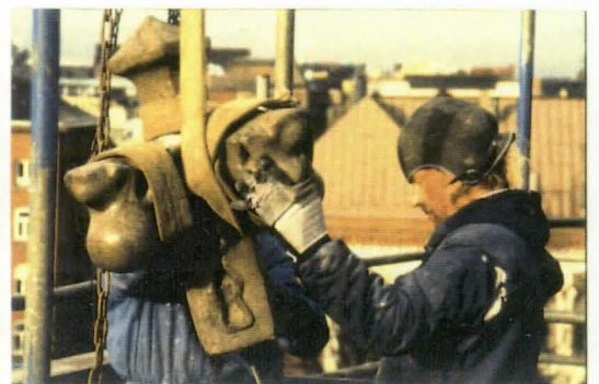
READJUSTING A FINIAL OF A SMALL PINNACLE.
