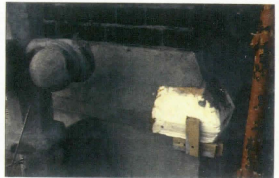
REPAIR OF (ANOTHER) CORNER. A DISPENSABLE MOLD IS USED.
