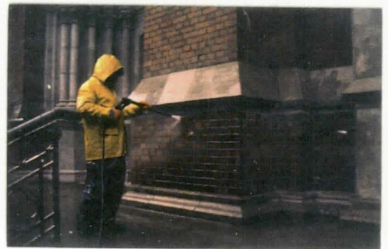
FLUSHING THE WALL WITH CLEAN WATER. THE REPAIRED SURFACES ARE VISIBLE,
