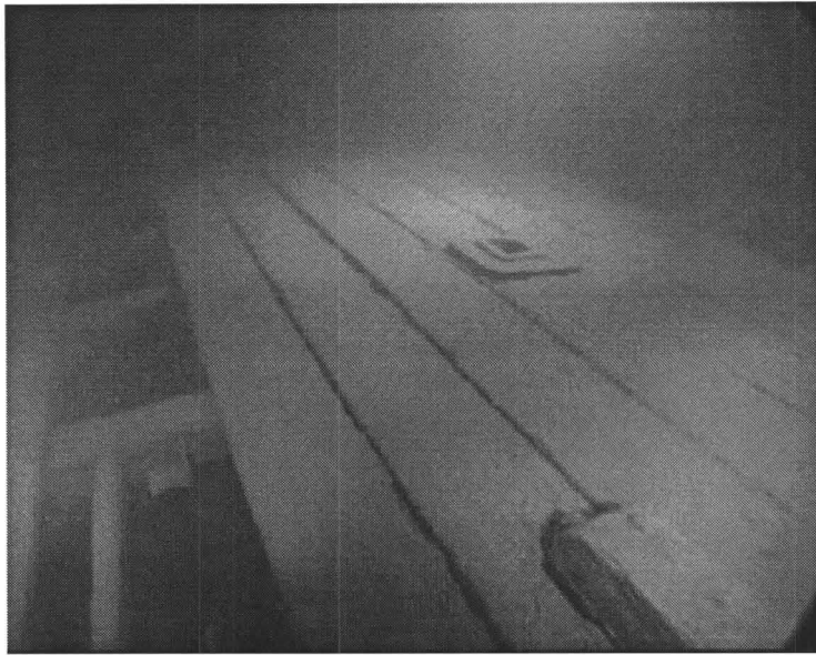
Picture 36. The poop deck viewed from the aft port side corner. A rectangular opening can be seen in the middle of the poop deck. A port side transom knee can be seen in the forefront. Photo by P. Raasakka & J. Kaasinen.
